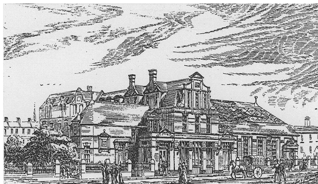
Bunhill Memorial Buildings, 1881, on Coleman (later Roscoe) Street
