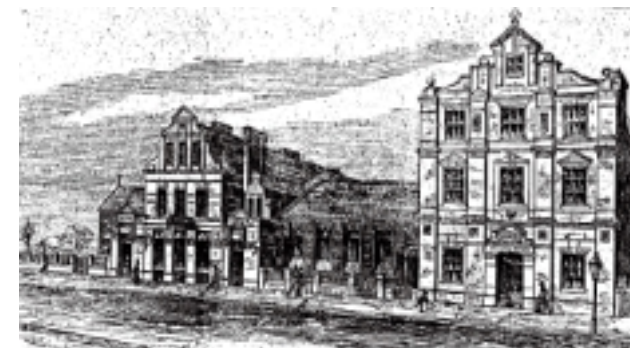
Bunhill Memorial Buildings, Showing the New Adult School Extension, 1888
